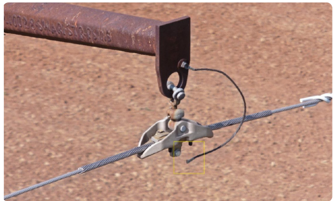
Ground wire disconnected from the overhead shield wire - SkySpecs' Horizon
